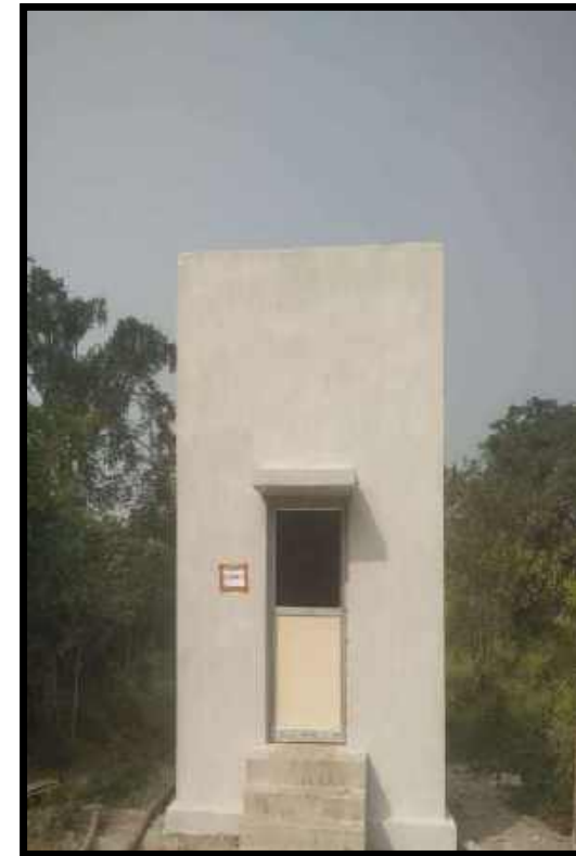
CAAQMS-3: Near DVC sub-station area.
